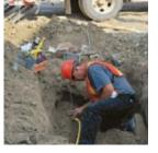
Traditionally during construction, gas lines are laid in one trench and utility wires are laid in an adjacent trench. This results in extra time and effort to schedule and coordinate more than one contractor. As well, because the additional contractor has to work beside a previously excavated trench, utility stakeouts are required.
